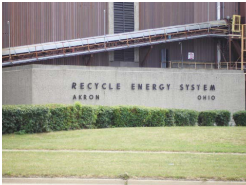
Akron Thermal Limited Partnership (RES Steam Plant entry)
